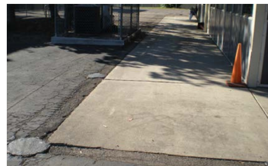
Paving in poor condition across campus.
