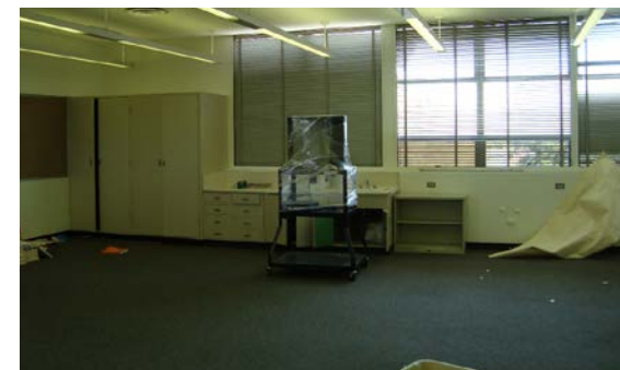
Standard modernization needed in classrooms.
