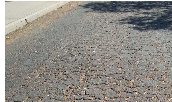
AC paving poor at parking lot.
