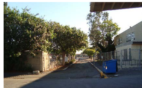
Drainage issues at the south of campus.
