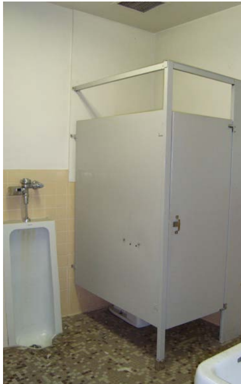
Provide ADA accessible restrooms.
