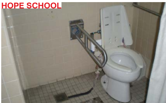
Additional specialized toilet facilities are needed.
