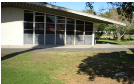
Landscape and irrigation in need of renovation.
